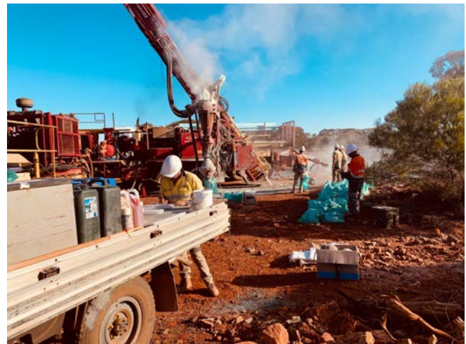
Sampling/Logging RC drilling Credo Well (March 2020)
